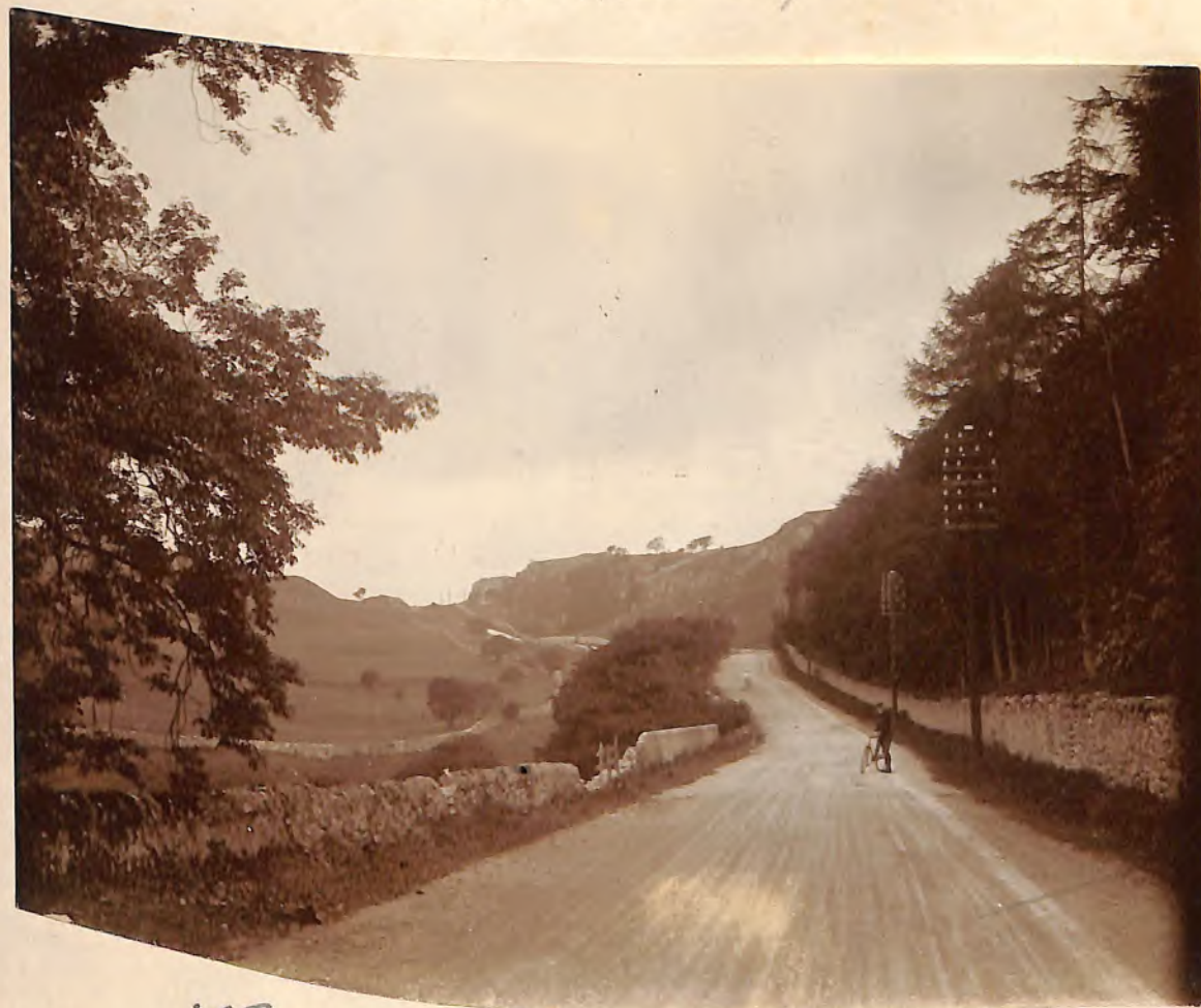
Road at foot of Giggleswick Scars.
