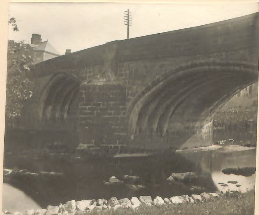
Old Ribbed Arches of Settle Bridge.
