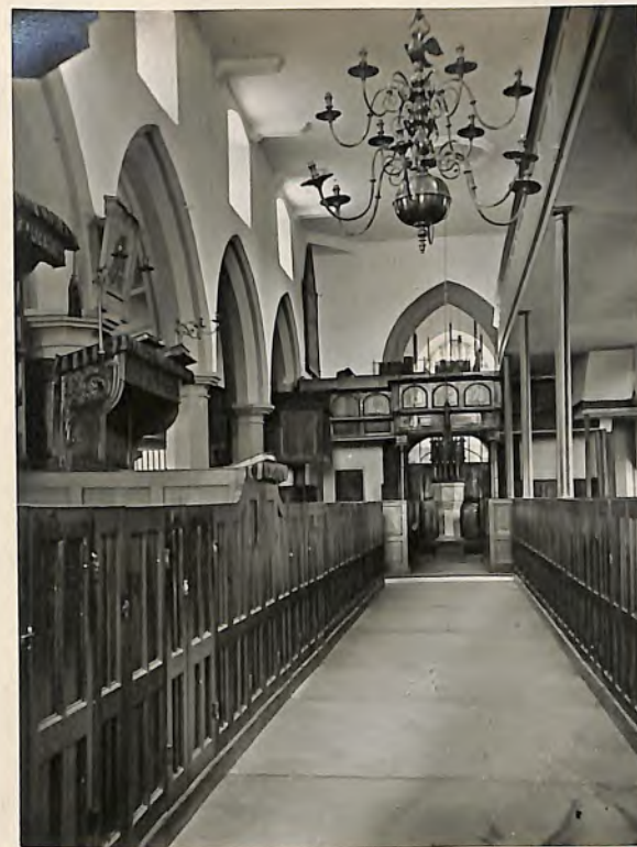
Giggleswick Church before restoration.
