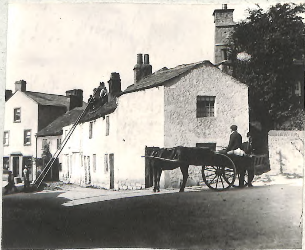
Cottages on "The Steps" in process of re-roofing, &c.
