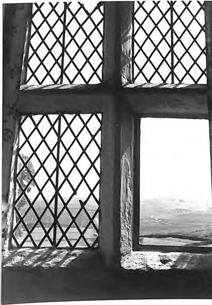
Window at Lodge Hall.
