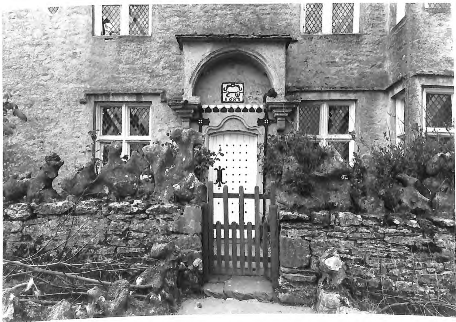
Front of house, similar size photograph in file.
