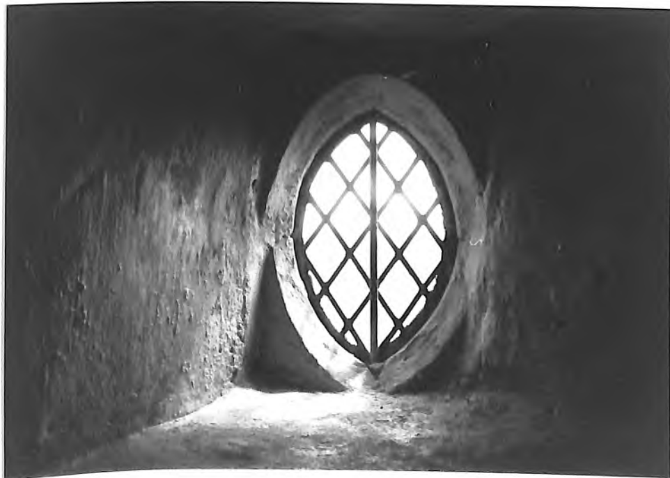
window at Lodge Hall.
