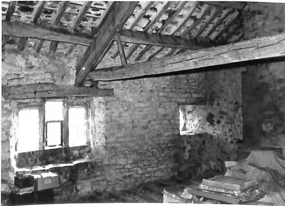
Window and attic at Lodge Hall.
