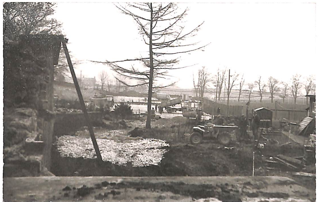
CONSTRUCTION BY SETTLE R.D.C.
