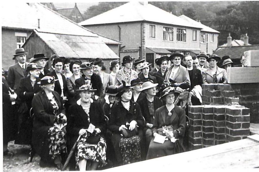
LAYING THE FOUNDATION STONES ON 5 JULY 1939 "SUNDAY" AT ST JOHN'S "SCHOOL" HALL
