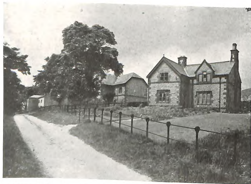
Cottages at Waterhouses showing Pt. Lot 1 in foreground and Pt. Lots 3 and 2 beyond
