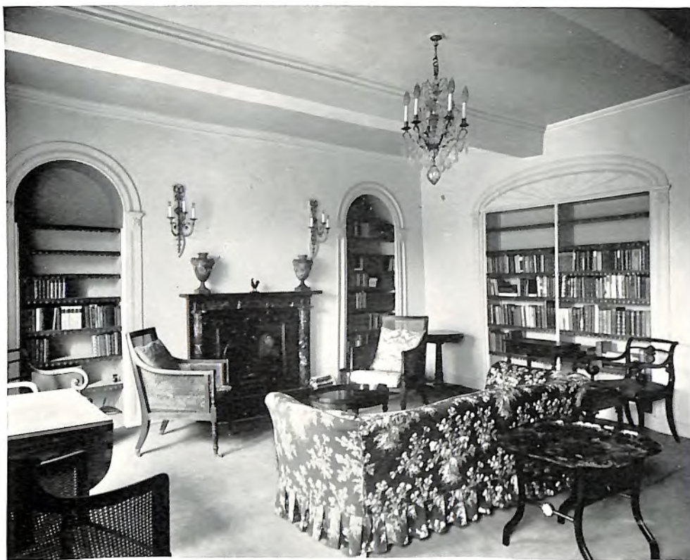
Eshton House—The Lounge
