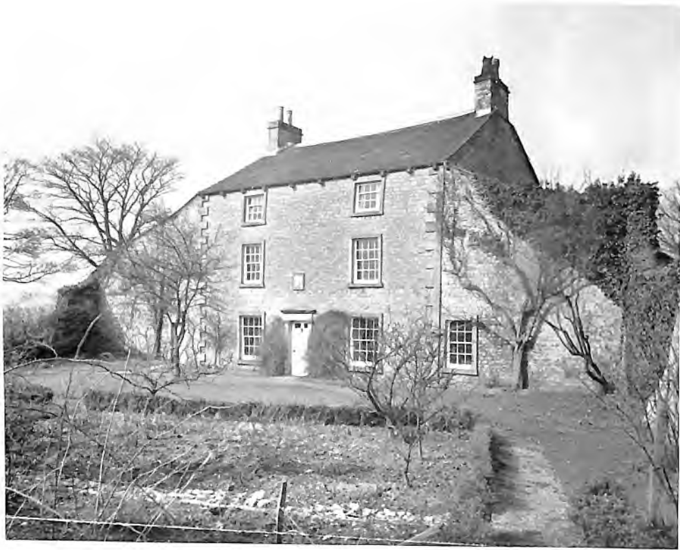
Eshton Grange Farmhouse (Lot 3)
